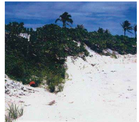
Detrital levee after construction with vegetation (source: M. Porcher)
