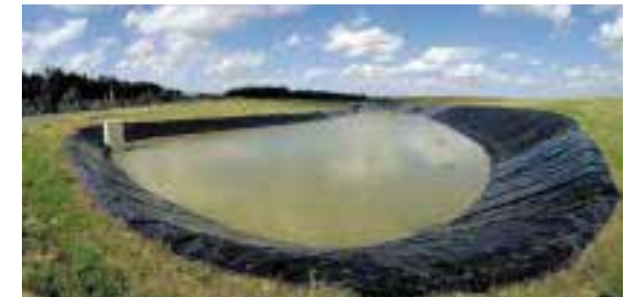
Retention basin at Angers-Marce Airport
