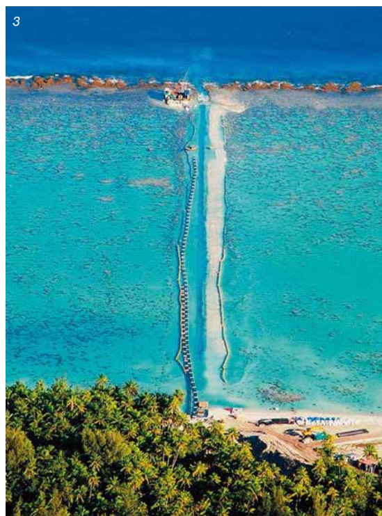
1: aerial view of Tetiaroa atoll and its pipe installation, 2: view of the underwater pipeline and its fixations, 3: aerial view of pipeline installation on the reef flat.
