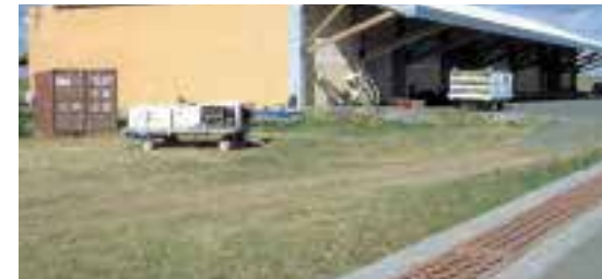
Dzaoudzi Airport (Mayotte): Drainage channel grate
