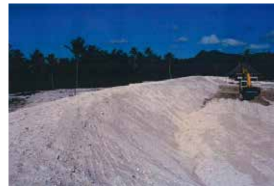
Artificial detrital levee under construction (source: M. Porcher)
