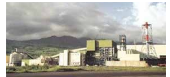
Gol coal-bagasse thermal power station. Source: ©Arer Mayotte report 2011
