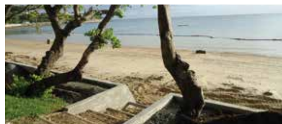
Noumea: Sloping wall along the Baie des Citrons coastal road
