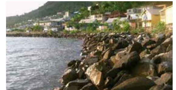
Medium sized rock protection – Chiconi, Mayotte. Photo: © Dem Boitcha
