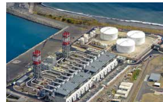
Thermal power station in Le Port, Reunion Island (source EDF)
