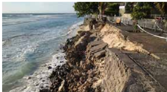
Collapsed beach seawall in Saint Paul, Reunion Island 2012. Photo: © BRGM
