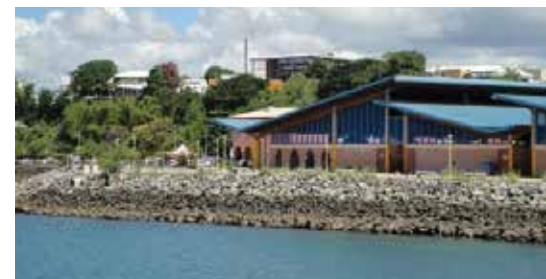
Mamoudzou: Medium sized rock embankment protecting the new market. Photo: Philippe Mathieu
