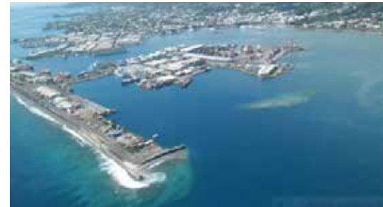
The port of Papeete - Large flood walls and rocks. Photo: © eminatetcie.canalblog
