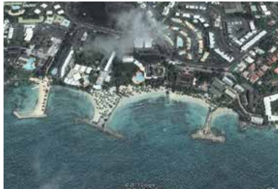
Gosier aerial view (Guadeloupe) - Beach Protection: groynes and breakwaters with medium sized rocks. © Google Earth
